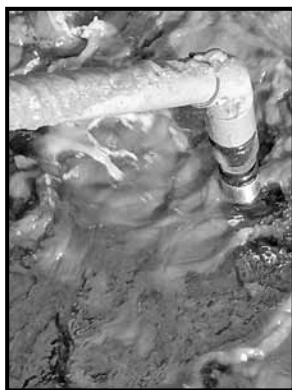
#5 & #6 Aerator Oxygen Sensor and Float Ball
