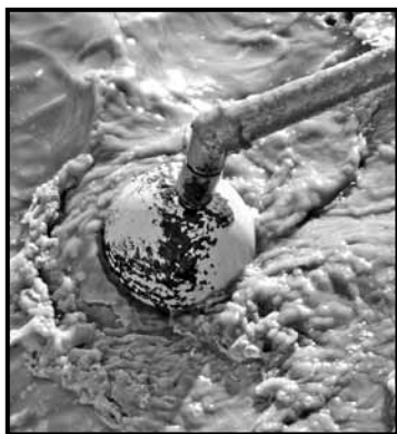
#5 & #6 Aerator Oxygen Sensor and Float Ball
