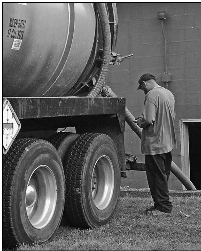
Removal of scum, grease and wipes from the Harmony Street Pump Station
