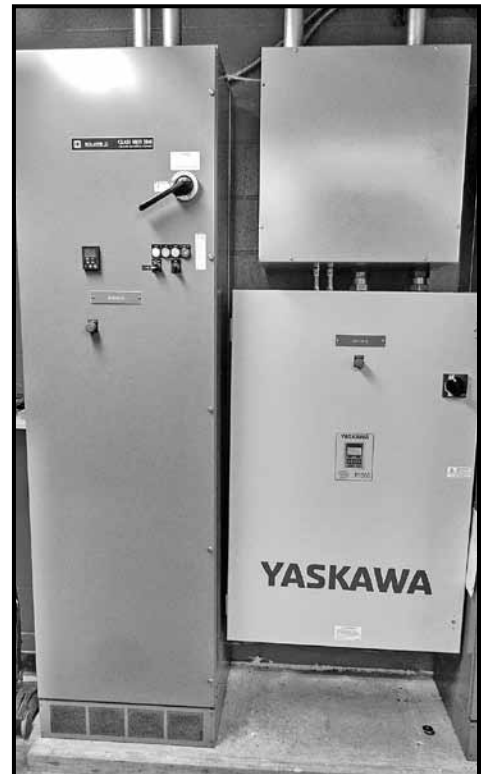
Left: New Variable Frequency Drive (VFD) for #2 Return Sludge Pump
