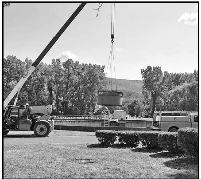
South Clarifier mechanical components being dismantled and removed.
