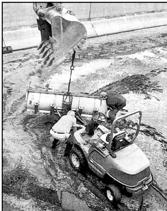
Above: Aeration Tank Cleaning
