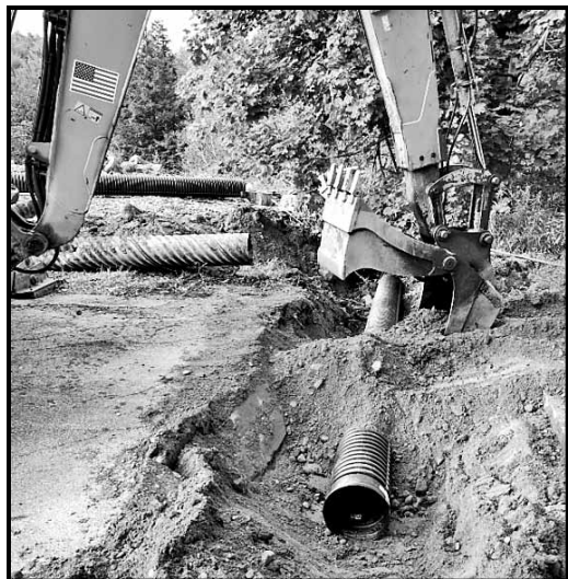
Above Right: Excavation and replacement of corroded pipe on Upper East Hoosac Street.
