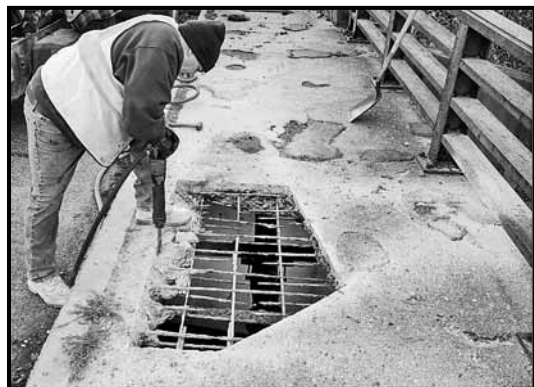
Above Left: Repair of deteriorated concrete walkway on the Spring Street Bridge.
