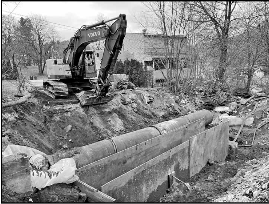
Left: Northern Construction, LLC of Palmer, Ma installing footings for a new box culvert on Davis Street.
