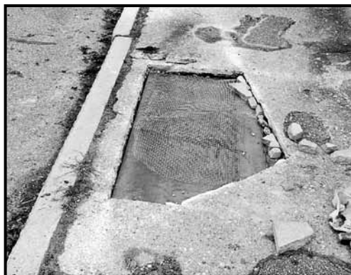
Above Left: Repair of deteriorated concrete walkway on the Spring Street Bridge.
