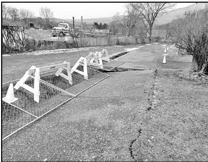
Collapsed culvert off of Jordan Street
