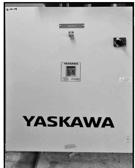
Newly installed equipment: Left & Center - Hypochlorite probes/sensors in contact channels; Right - VFD for #4 Aerator
