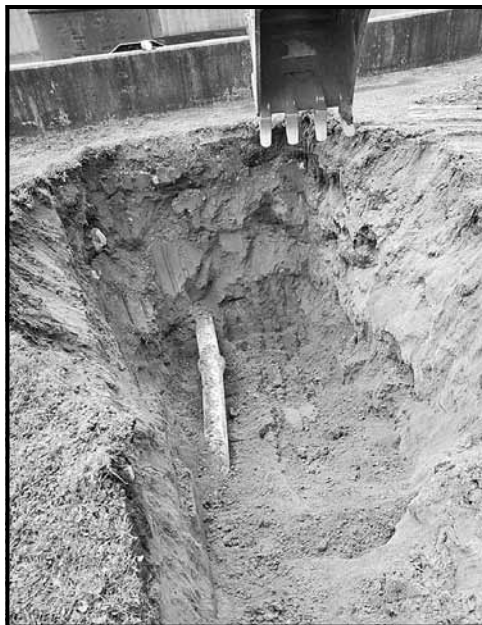
Above & Below: Installation of new piping and shut-off valve from south clarifier
