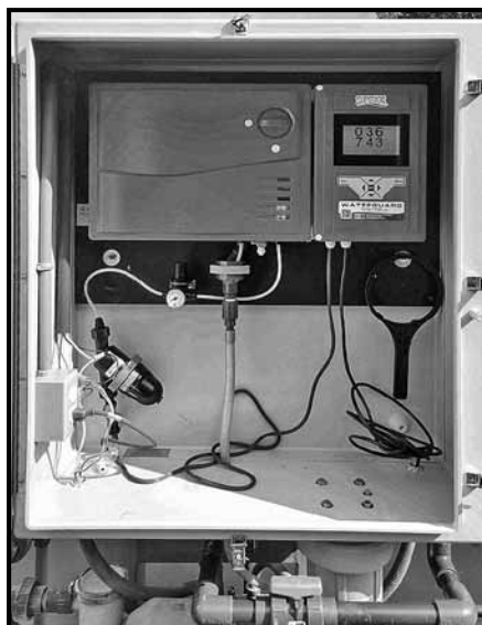
Newly installed equipment: Left & Center - Hypochlorite probes/sensors in contact channels; Right - VFD for #4 Aerator
