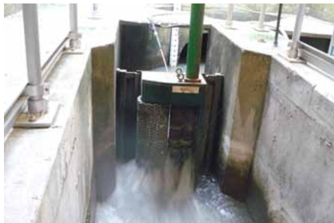
Channel Grinder located in influent wet well
