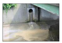
The effects of upstream erosion and sediment transport observed at a stormwater discharge to the Hoosic River at Spring Street.
