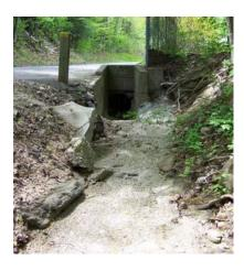
This site is a drainage swale along Glenn Street that is partially lined with concrete before it enters a 32" pipe that eventually discharges to the Hoosic River.
